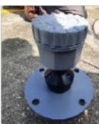
The ultrasonic level gauge and overfill prevention alarm device installed in the toluene storage tank
